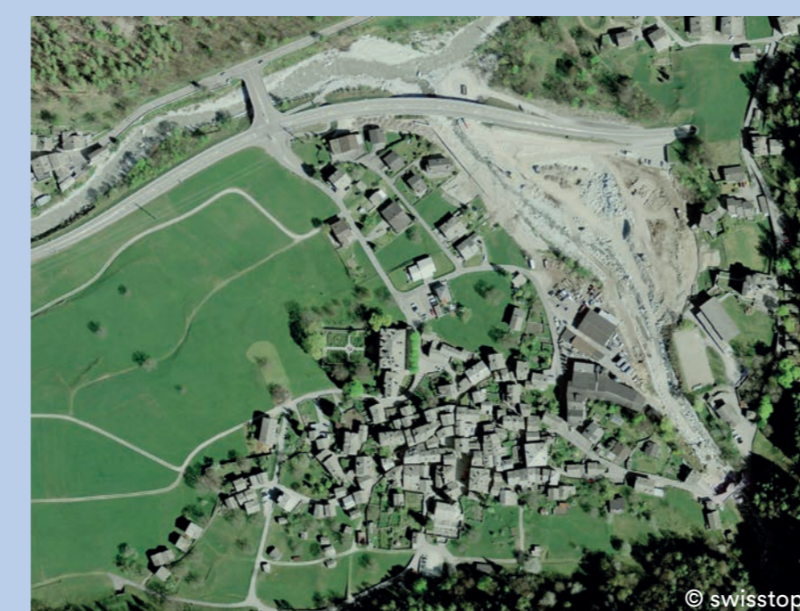
Bondo, 2015 ("Bondo I" under construction)
